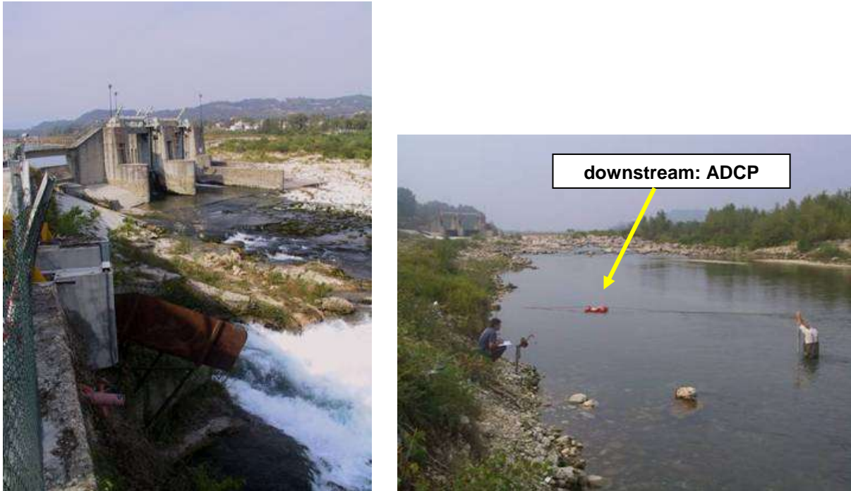
Figure 21: MIF measurements just downstream Nervesa dam (Piave River)
