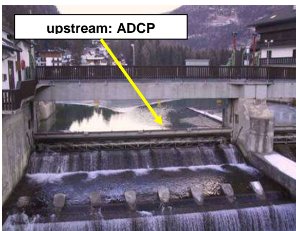
Figure 20: MIF measurements at Alleghe dam (Cordevole River)
