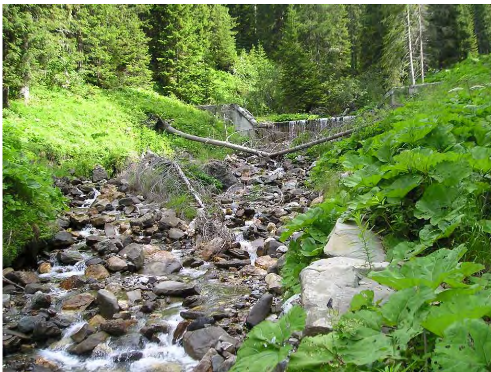
Figure 77: check dams along the channel reach downstream the withdrawal point
