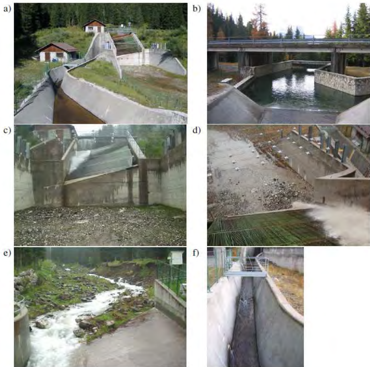
Figure 68. Rio Cordon measuring station: a) Downstream view of the bedload storage, the outlet flume and the two buildings hosting instrumentations and the emergency power system; b) Upstream view of the fine sediment settling basin; c) Downstream view of the separating grid, the bedload storage area and the cable frame which host the 24 ultrasonic sensors; d) Upstream view of the bedload storage area; e) Downstream view of the inlet channel; f) Downstream view of the outlet channel. (From Mao et al., 2010)
