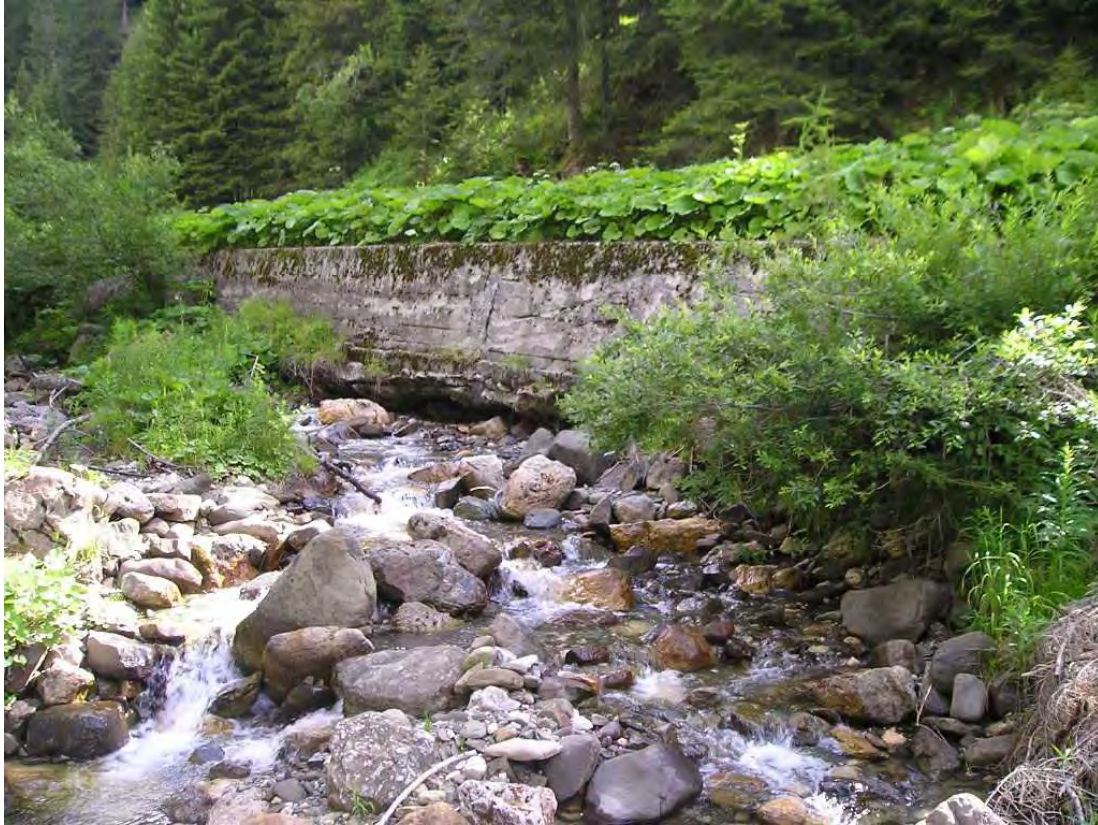
Figure 78: check dams and lateral bank protection works along the channel reach downstream the withdrawal point
